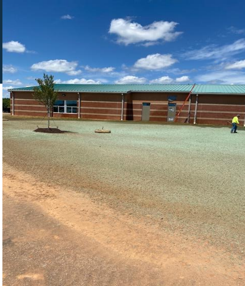
Classroom Wing Exterior
