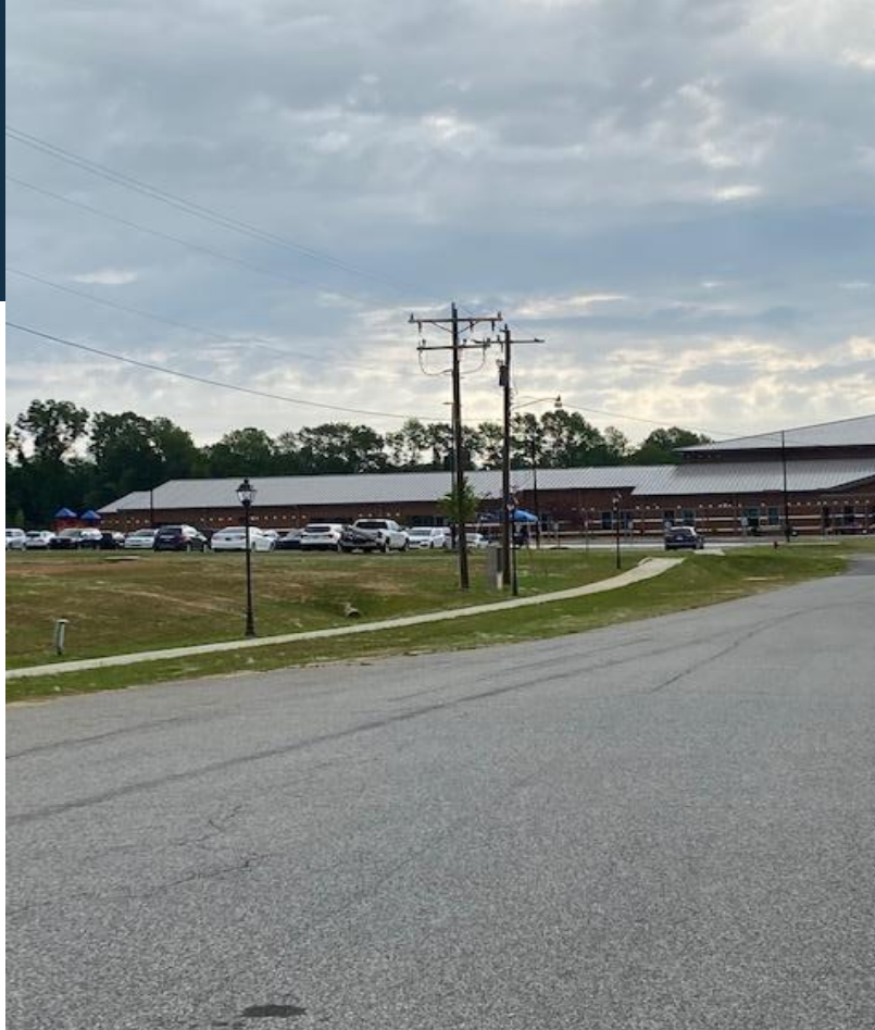
Sidewalk and Lights
